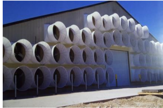
Figure 3: A typical ventilation system in ECH system
